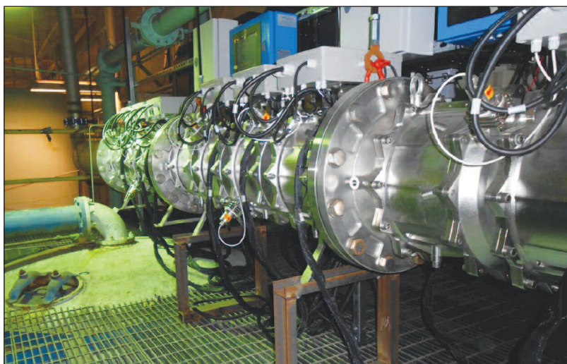
Figure 4: System installed at a 3 160 MW coal-fired power station for evaluation.
