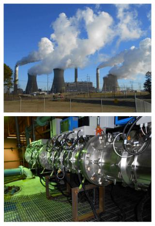
Incorporating HOD<sup>™</sup> UV at Plant Bowen has reduced the use of SMBS for dechlorination and minimized the frequency of micron filter replacement.
