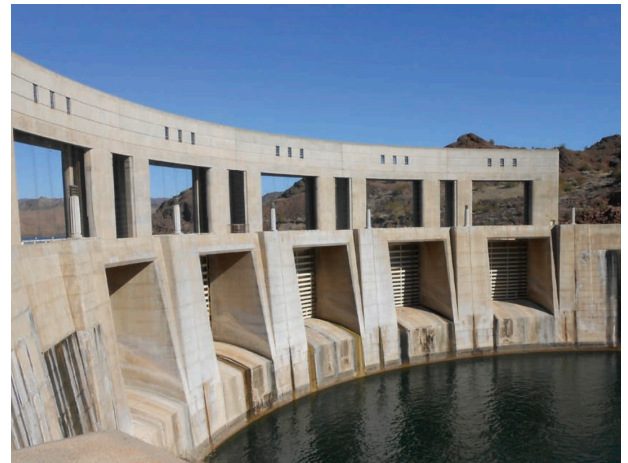
HOD UV systems were installed at Parker Dam to address biofouling concerns from Aquatic Invasive Species (AIS).
